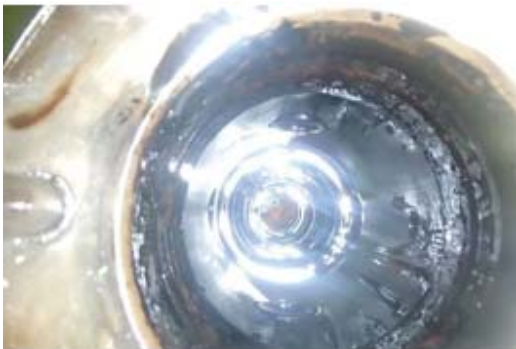
写真-3 Pump Housing Barrelを抜いた状態 Photo-3 Pump Housing with Barrel Removed
